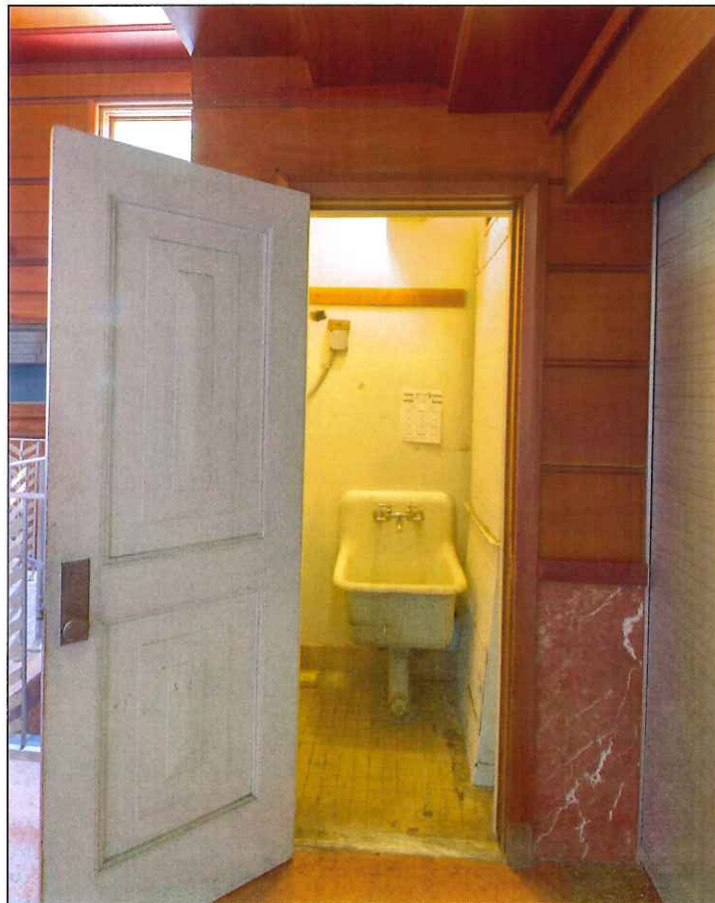
Image 16: Janitor's closet in lobby (Schafer, 2016)
