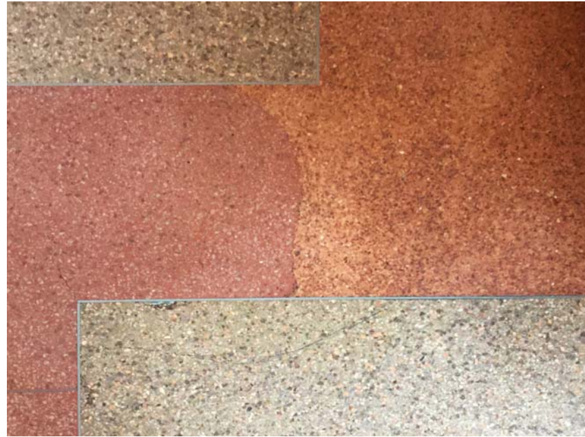
Terrazzo patch at location of former entry vestibule
