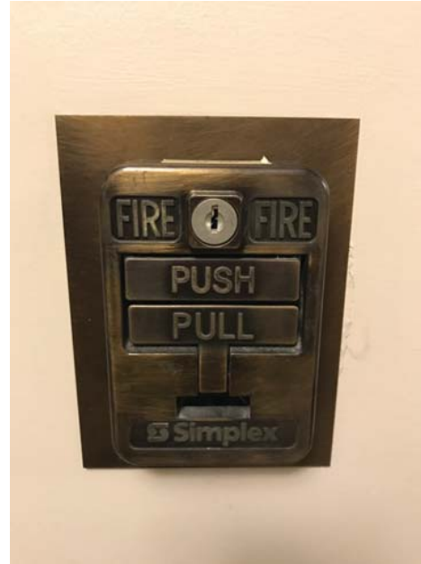
PULL STATION (COLOR TO BE BRONZE OR RED) NOT TO SCALE
