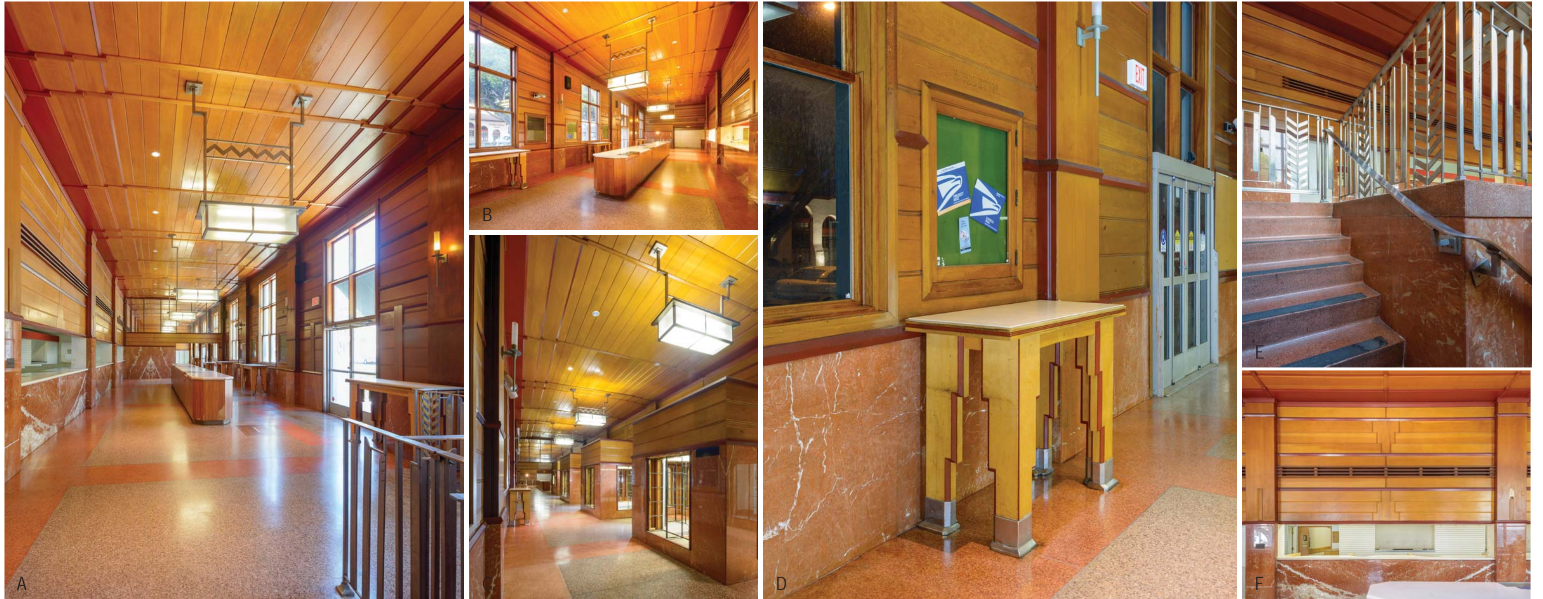
A. Southern portion of lobby with service counters, looking North. B. Southern portion of lobby, looking South. C. Northern portion of lobby with postal box alcoves, looking South. D. Historic lobby table and bulletin board E. Terrazzo stairs, curved stainless steel handrail and railing from landing F. Detail of Lobby service counter bay
