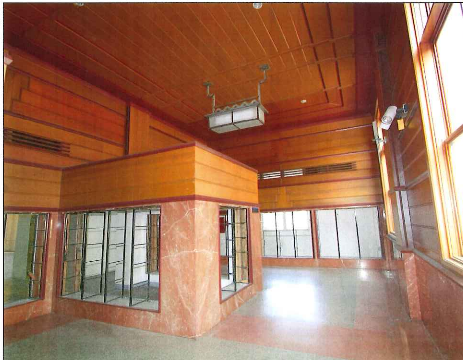
Image 10: Northern portion of lobby, looking north, added projecting postal box alcoves and altered north wall and truncated historic light fixture visible (Chattel, 2014)
