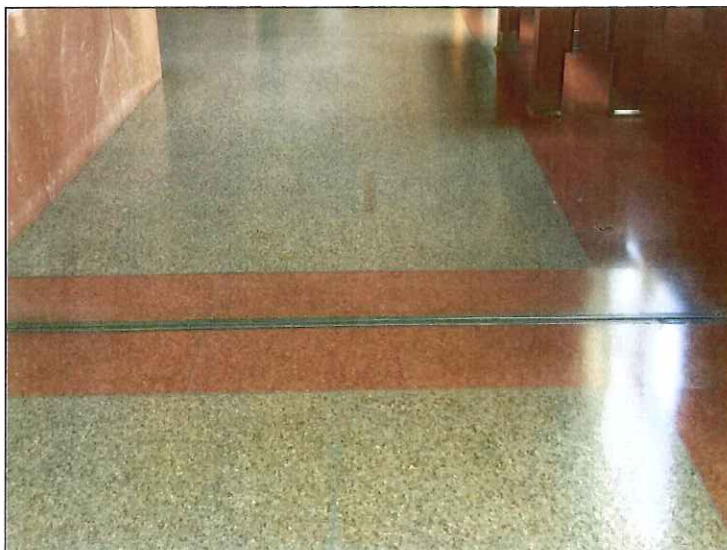
Image 27: Existing floor conditions - Channel through terrazzo border at existing dividing wall (Waisler, 2016)
